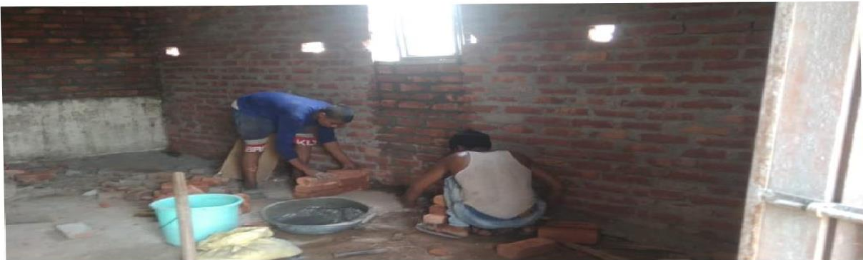
NEW STORE ROOM UNDER CONSTRUCTION
